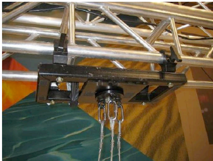
Figure 2 - Swivel Plate, pictured while attached to 12" box truss
